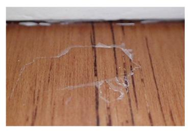
Floor finishes peel because the floor was contaminated or improperly prepared when the finish was applied.
